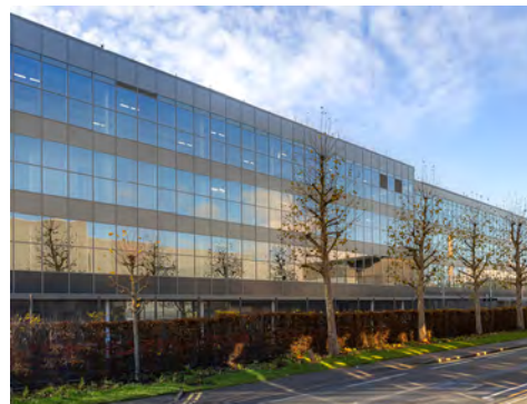
Recent data centre development on Slough Trading Estate, UK
