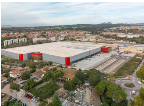
SEGRO Logistics Park Cerdanyola, Spain
